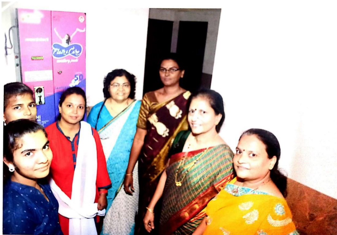
Installation of Sanitary Napkin Vending Machine & Incinerator (23/07/2018)
